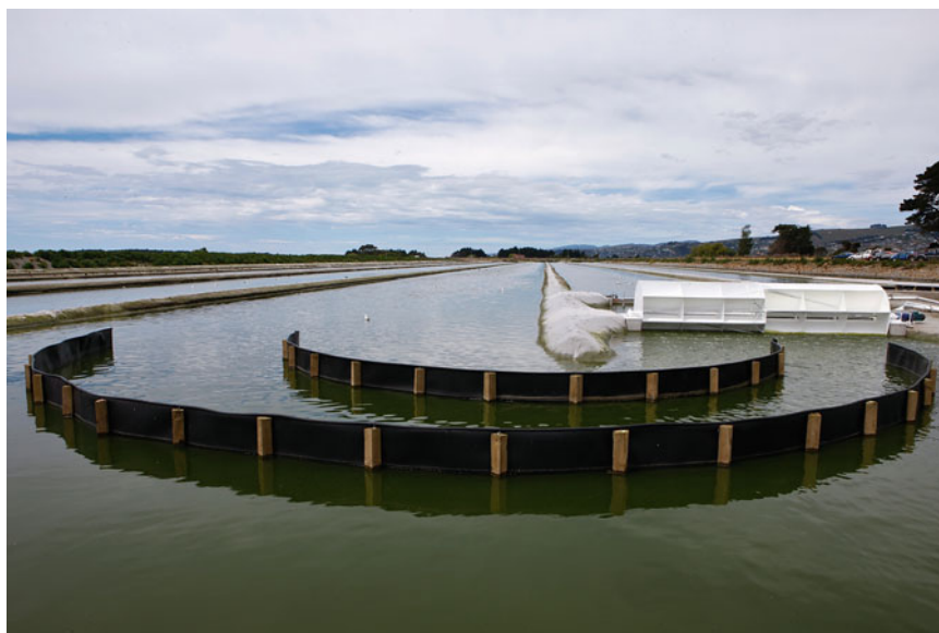
Fig. 9.3 One of the four wastewater treatment HRAP (1.25 ha) with CO 2 addition at Christchurch, New Zealand
