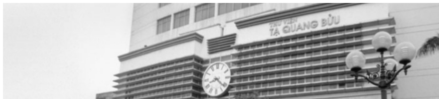
Ta Quang Buu Library, Hanoi University of Science and Technology. Location of VIASM
