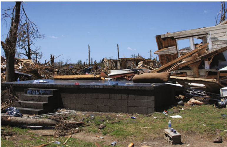
Residential damage in Tuscaloosa, Alabama, from the April 27, 2011 tornado outbreak.
