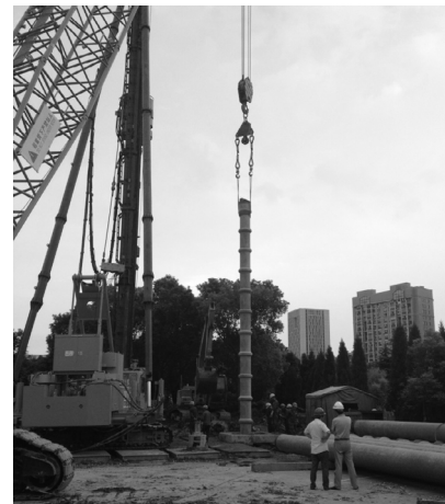
Fig. 5 Test pile installation
