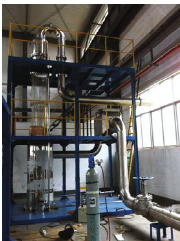
Fig. 16 Test platform under construction for structured packing performance by Hangyang
