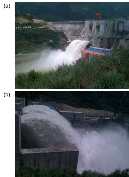
Fig. 1 Flood discharge with ski-jump flow of Wudu dam spillway in China
