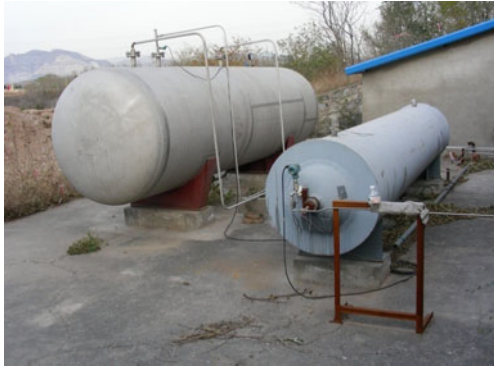
Fig. 2 Installation of the fatigue test system
