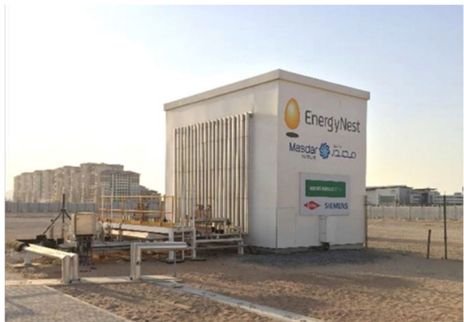
Fig. 9 Photograph of fully commissioned EnergyNest thermal energy storage with 4 \times 250 \text{ kWh}_{\text{th}} capacity at Masdar Institute Solar Platform, United Arab Emirates [103]
