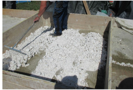
(a) Half of the sand is spread on the ground and covered with crushed quicklime. The volume ratio of quicklime to sand is 1:7-9.
