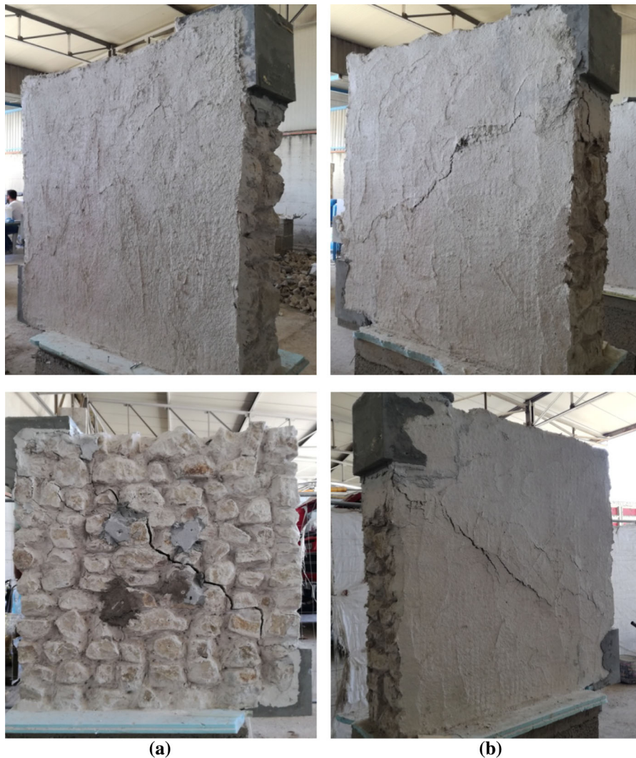
Fig. 5 FRCM strengthened panels: crack pattern at failure for a single-side configuration and b double-side configuration
