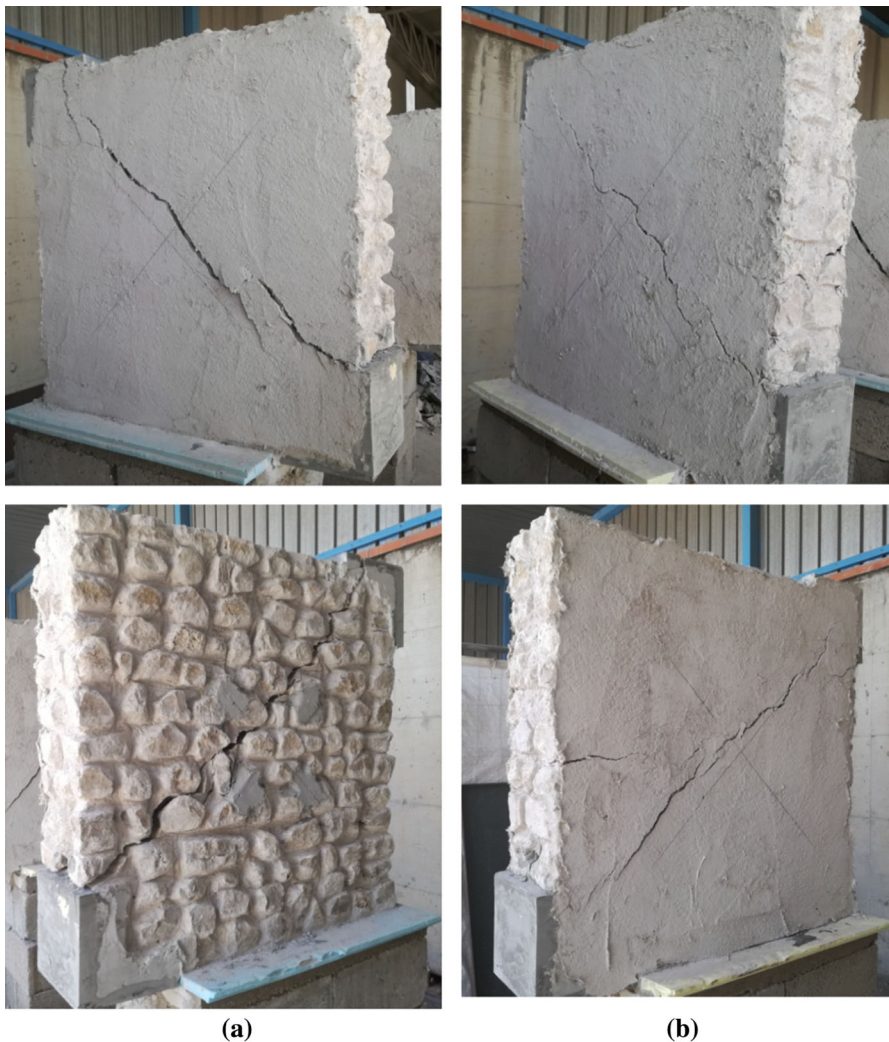
Fig. 9 FRM-B strengthened panels: crack pattern at failure for a single-side configuration and b double-side configuration
