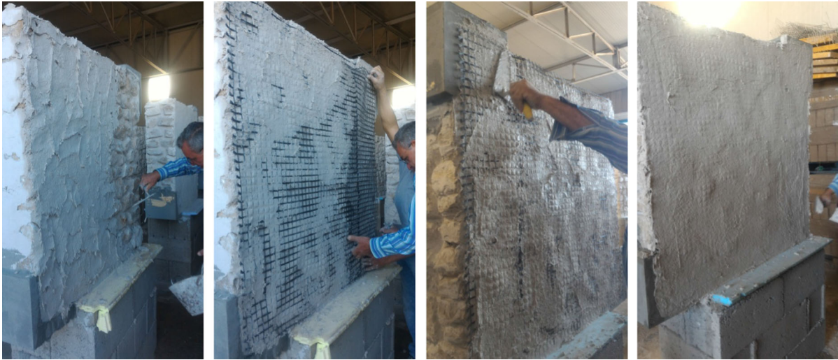
Fig. 2 Strengthening procedure for FRCM technique
