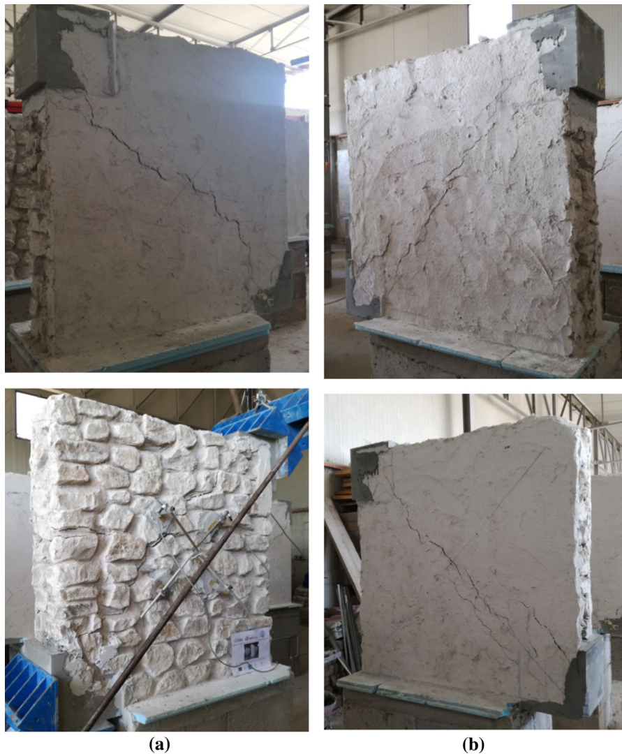
Fig. 7 FRM-A strengthened panels: crack pattern at failure for a single-side configuration and b double-side configuration
