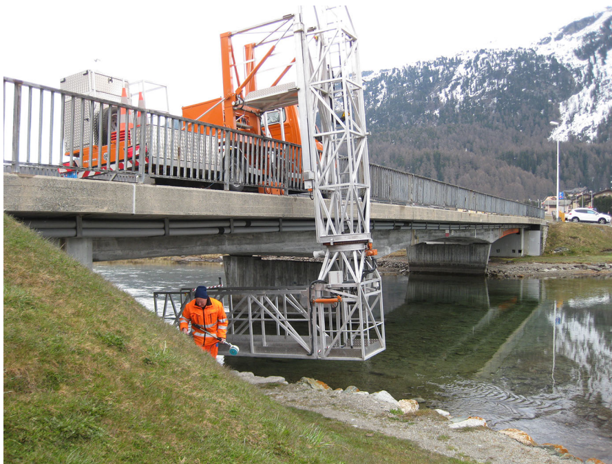
Fig. 6 Example of the inspection (here: potential mapping) of the underside of a bridge girder, illustrating that costly equipment and laborious procedures are needed to perform the measurements on the concrete surface of interest. This is one of the main factors driving the costs of condition assessments.
