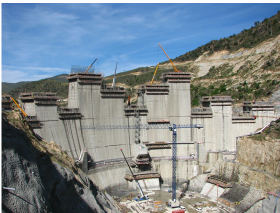
Fig. 4 Baixo Sabor dam during construction
