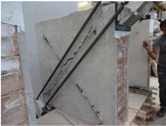
Fig. 7 Reinforced panel after failure (panel reinforced with mortar Type D)
