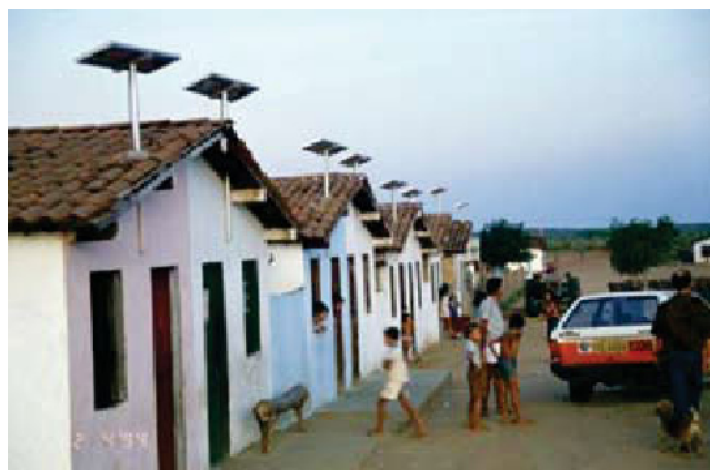
Figure 1. In the village of Irapura, Ceara, Brazil, homes were fitted with 50 W solar panels for night lighting, television, and radio. A battery stores electricity generated by the solar panel for use at night. (Photograph by Roger Taylor.)
