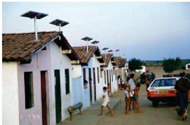
Figure 1. In the village of Irapura, Ceara, Brazil, homes were fitted with 50 W solar panels for night lighting, television, and radio. A battery stores electricity generated by the solar panel for use at night. (Photograph by Roger Taylor.)
