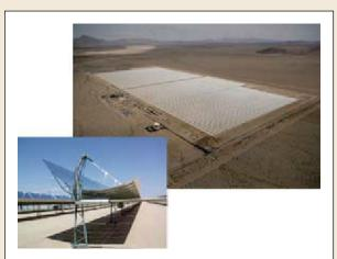
**Figure 1.** Aerial photograph of Acciona's Nevada Solar One, a 64 MW parabolic trough power plant near Las Vegas, Nevada, that covers 280 acres (*Credit:* Acciona Solar Power). Inset: Closeup of an individual parabolic trough unit at Kramer Junction, California, showing the curved mirror and the receiver (*Credit:* Henry Price).
