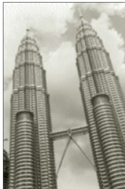
Figure 3. Petronas Twin Towers in Kuala Lumpur, Malaysia, the tallest-structure worldwide, uses concrete instead of steel as the material for the column. Courtesy of the Embassy of Malaysia.
