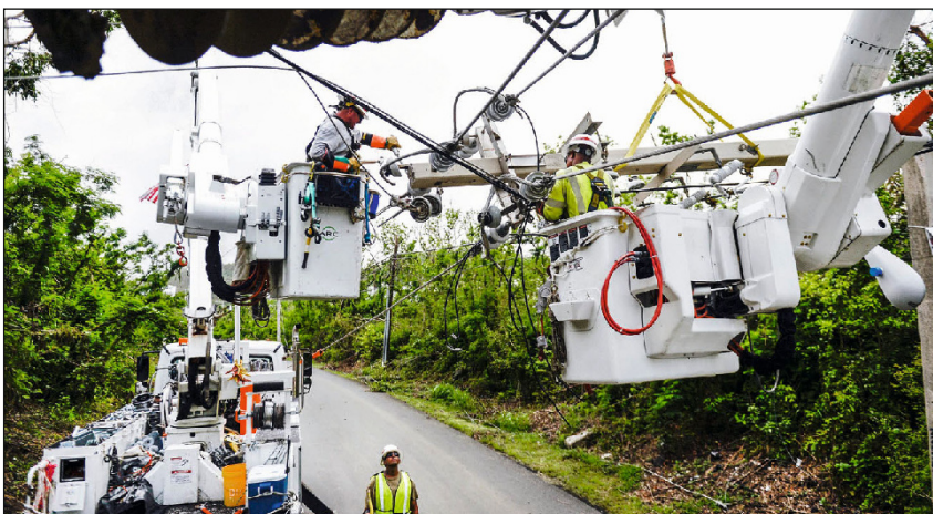
Transmission and distribution specialists assigned to Company D, 249th Engineer Battalion (Prime Power) of the US Army Corps of Engineers, repair power lines in Rio Grande, Puerto Rico, after Hurricane Maria. Photo credit: Master Sgt. Joshua L. DeMotts, US Department of Defense.
