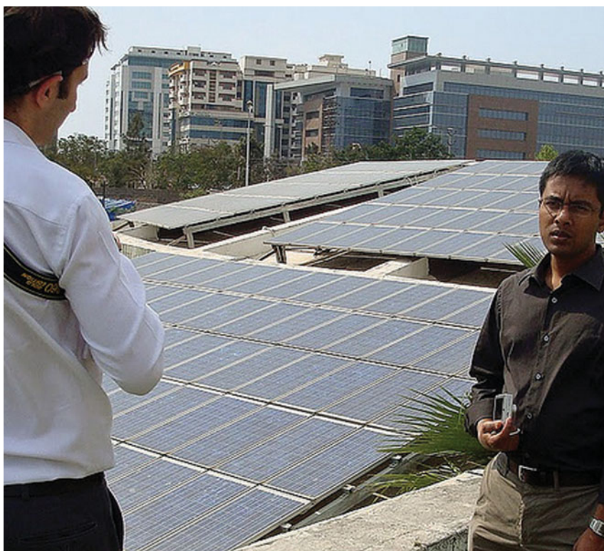
Solar panels on the roof of the Confederation of Indian Industry's Godrej Green Business Center in Hyderabad. Credit: Natural Resources Defense Council
