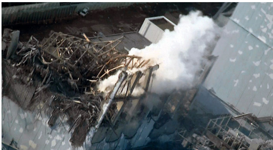
A picture taken from a helicopter on March 16, 2011 of an explosion caused by a build-up of hydrogen in the Fukushima Daiichi Unit 3 nuclear power station in Japan. Although the reactor's primary containment vessel was not damaged, the explosion injured 11 people. Credit: Tokyo Electric Power Co.
