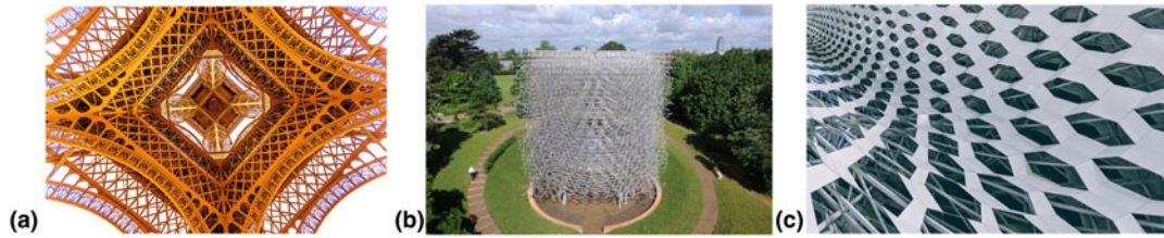
Figure 2: (a) Upward view of the Eiffel Tower in Paris, showing hierarchical structure of 18,000 iron parts (mostly struts) connected with 250 million rivets. 59 (b) The Hive , installed in London's Kew Gardens in 2016, simulates a living beehive. Its lattice, 17 m in height, comprises 170,000 aluminum struts and connectors. 60 (c) A view inside the Bao'an airport at Shenzhen, with a 450,000 steel member structure allowing for high earthquake loads, with cross bracings providing high stiffness 61 (photo courtesy: Prof. J. Huang, Northwestern University, IL, USA).
