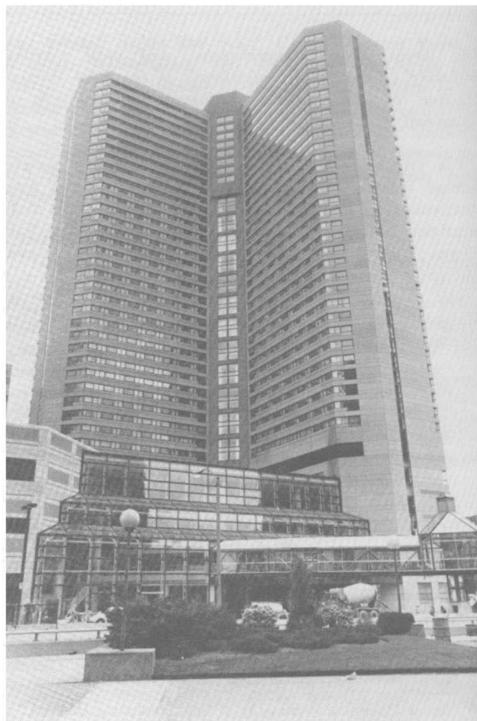
BOSTON MARRIOTT/COPLEY PLACE, rising 38 stories above the heart of the city, has the finest facilities for the expanded 1984 Annual Meeting of the Materials Research Society
