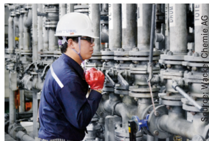
An employee supervises the production processes in the control room of the VAE plant in Ulsan. Wacker already produces VAE dispersions in South Korea for the adhesives industry.
