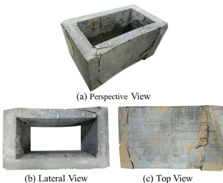
Fig. 15 Crack pattern for confinement specimen G02-S02-VCO
