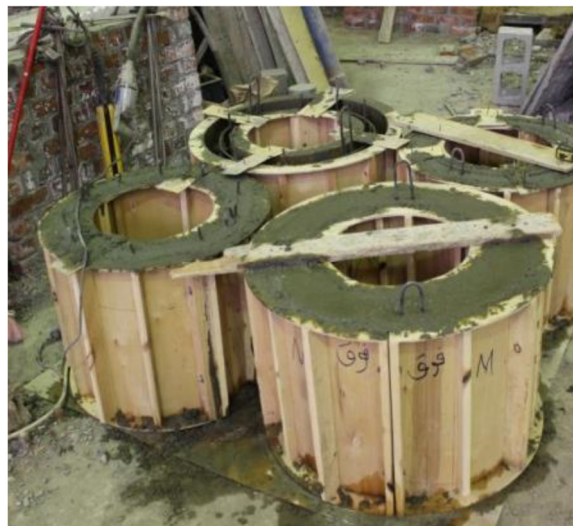
Fig. 5 The concrete casting of pipes
