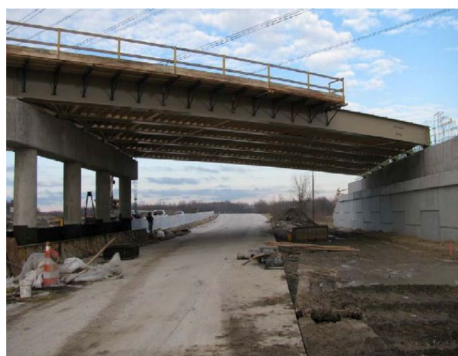
a) Michigan skewed bridge (Located at US)
