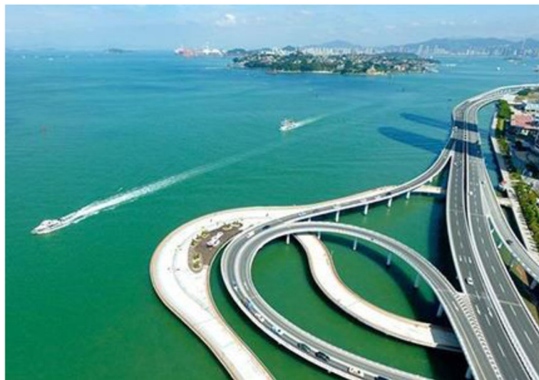
Fig. 1 A typical multi-span coastal bridge at southeast coastal region of China
