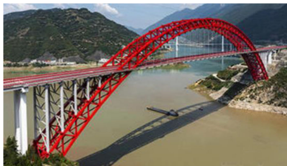
Fig. 7 Zigui Yangtze River Bridge
