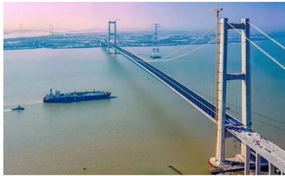
Fig. 4 Nizhou viaduct of the Nansha Bridge
