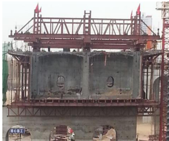
The PC box bridge girder on the pier top
