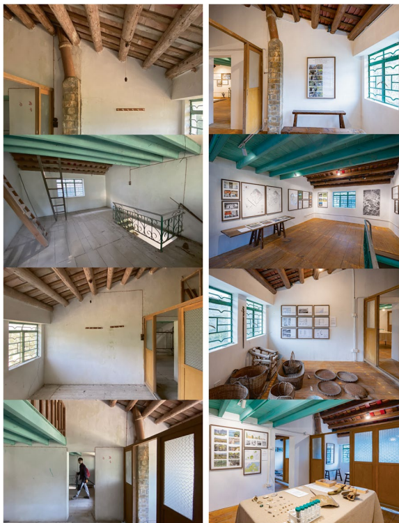
Fig. 9 Yeung House before restoration (left) and after restoration (right) (Source: the author)
