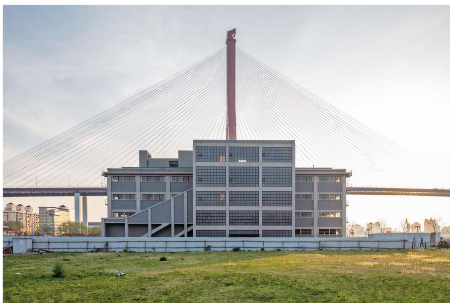
Fig. 19 West Elevation of the west wing after renovation (Source: Fangfang Tian)
