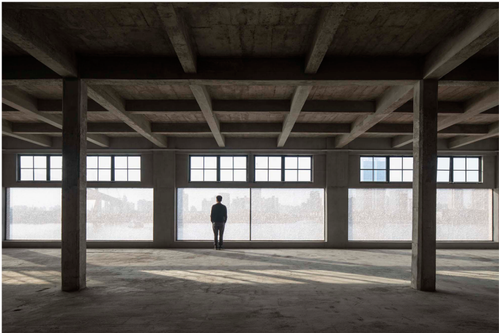
Fig. 11 Internal view of the façades made of screen-printed glass (Source: Fangfang Tian)
