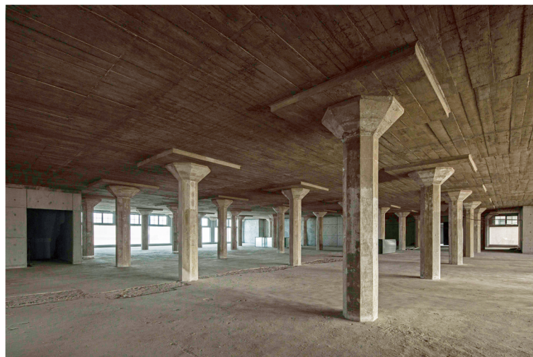
Fig. 9 Renovated beamless structural system of the interior (Source: Tianzhou Yang)
