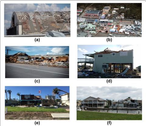
**Fig. 2** (a) Damage in Tyndall Air Force Base after Hurricane Michael, (b) St. Maarten after Hurricane Irma, (c) Grand Isle, LA after Hurricane Ida, (d) Damage in Holiday Beach Community, (e) Structural damage from Hurricane Harvey, and (f) Different response of two adjacent buildings in Rockport, TX
