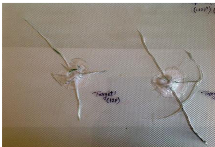
Fig. 3 Multiple fracture on the glass pane
