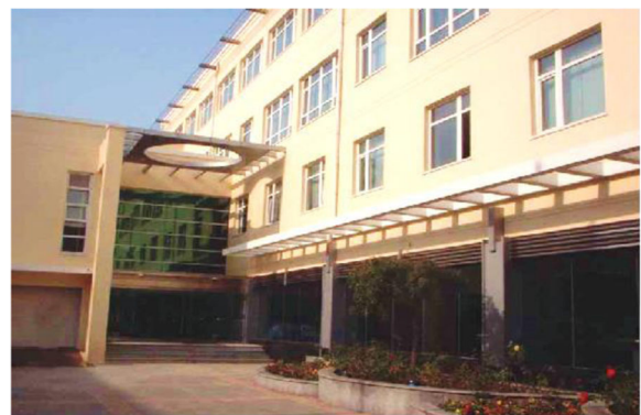
Fig. 8 Office building of the Tianjin Meijiang ecological community
