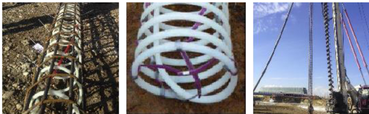
Fig. 21 Spiral borehole heat exchanger [16]
