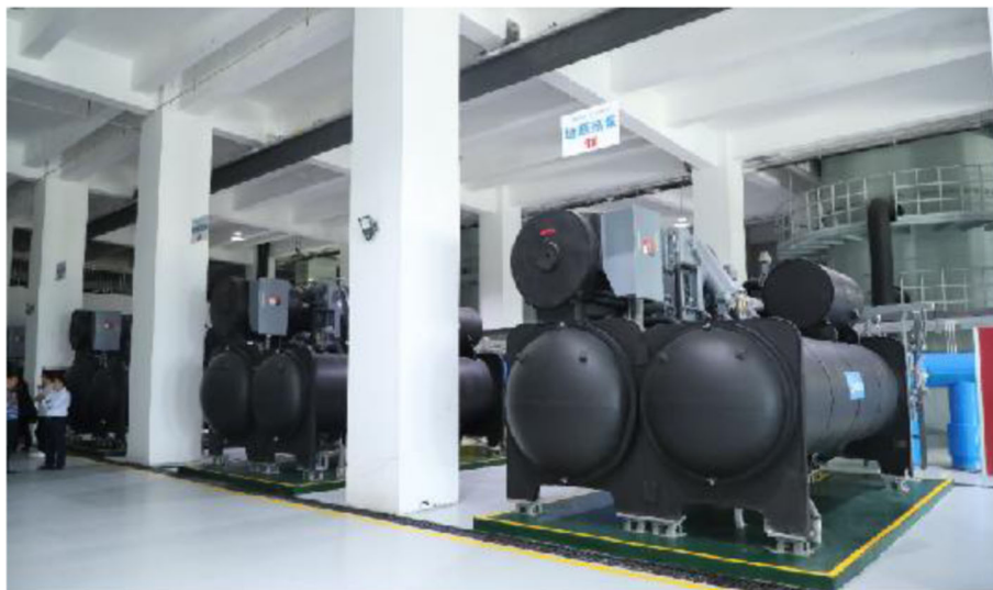
Fig. 14 Full falling film variable frequency centrifugal heat pump units
