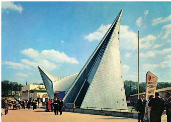
Fig. 10 Philips pavilion was a World's Fair pavilion designed for Expo 1958 in Brussels by the office of Le Corbusier. The building, which was commissioned by the electronics manufacturer Philips, was designed to house a multimedia spectacle of sound, light and projections celebrating post-war technological progress. Iannis Xenakis was responsible for much of the project management. [Figure copyright Wikimedia Commons: Wouter Hagens]
