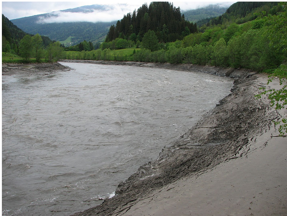
Fig. 13 Photograph of a bank of the Bodendorf reservoir during flushing
