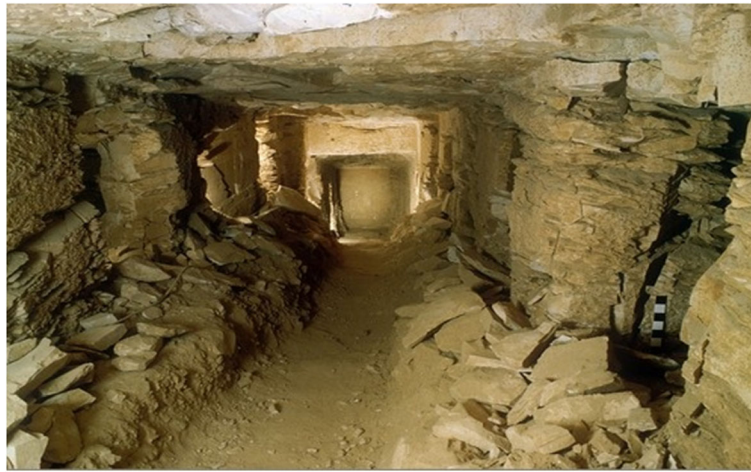
Fig. 9 Brittle rock, high stress conditions. Rockbursting (the sudden release of stored strain energy) bursts manifest themselves through sudden. (After TMP)
