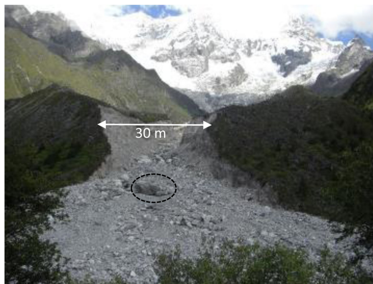
Fig. 5 Frontal view of the typical V-shaped channel morphology after the breach. A large dislodged boulder can be seen in front of the breached section
