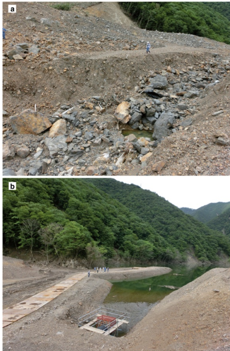
Fig. 1 a Exposed section of the materials composing the Akatani landslide dam b Upstream side of the Akatani landslide dam showing water inflow into the dam through an artificial drainage pipe. Note: People for scale (photo by Wang FW)
