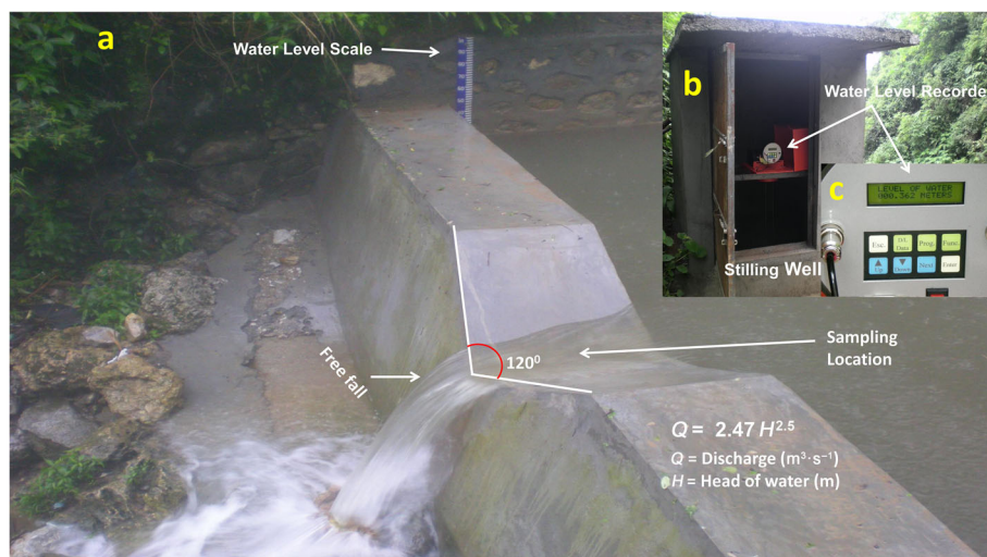
Fig. 2 View of the type of broad-crested compound weirs used to gauge streamflow at Arnigad and Bansigad
