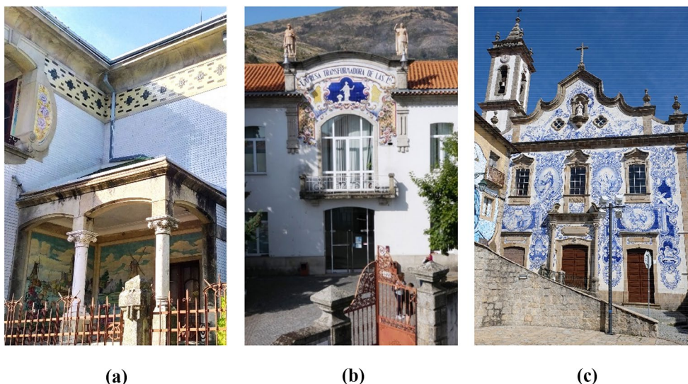
Fig. 2 a Residential building 'Palacete do Jardim', by architect Ernesto Korrodi (1915); b Industrial building 'Empresa Transformadora de Lãs', currently the Faculty of Engineering of the University of Beira Interior, by architect Ernest Korrodi, covered with Aleluia factory tiles (1920); c Religious building 'Church of Santa Maria Maior' (1886), covered with tiles from the Aleluia factory in 1943
