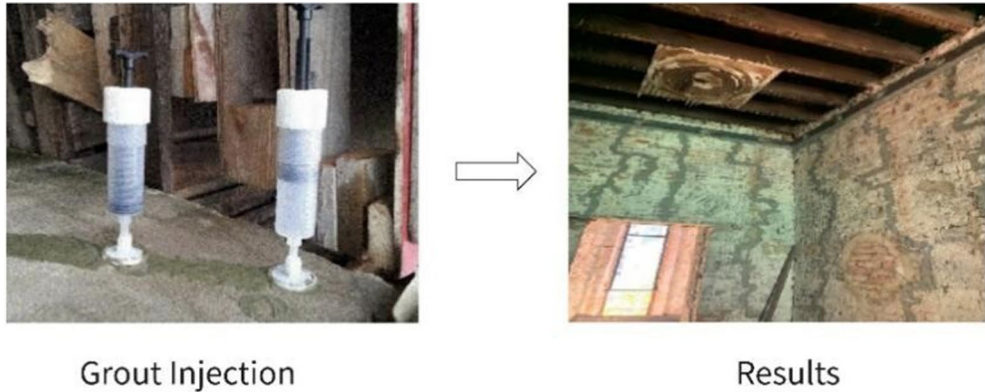
Fig. 20 On-site restoration techniques
