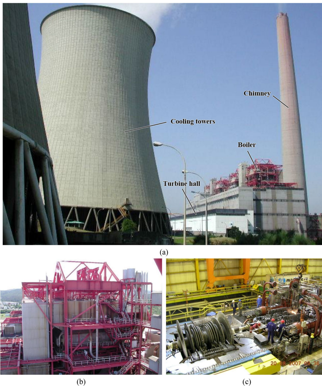
Fig. 8 a General view of the As Pontes power plant elements shortlisted for preservation. Details of the b boilers and c turbine hall
