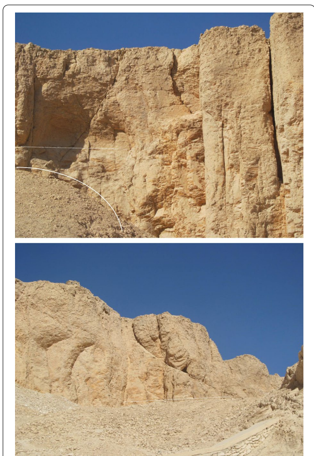
Fig. 15 Evidence of flash flood related erosion in the Esna Shale and vertical fissures in Unit 1 of the Thebes Limestone, delineation of the abandoned Excavations and its causeway. The subvertical wall-cuts were dug in the upper part of the Esna Shale Formation and at the base of the Thebes Limestone Formation. White arrows point to erosional gullies in the lower part of unit 1 of the Thebes Formation, in the Hanadi Member (Esna Shale Formation) and in the debris that cover the Esna Formation. Note that the gullies at the base of the Thebes Limestone and just below are commonly hollowed out, in particular on top and below the prominent base of Unit 1. These are probable evidence of flash floods. fallen blocks; unstable columnar block and open vertical fissures; screes. screes resulting from archeological excavations
