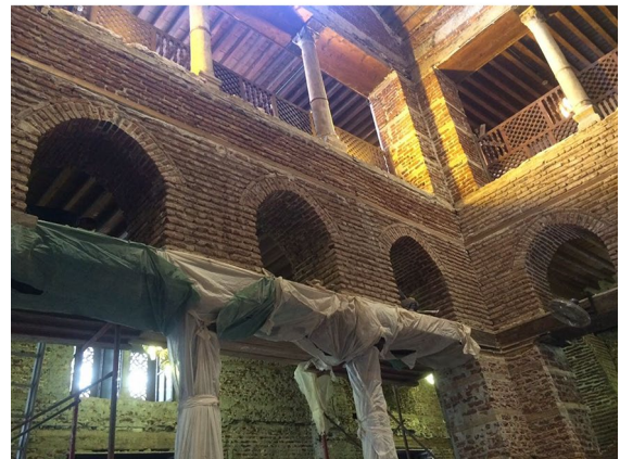
Fig. 21 The strengthening of the structural twelve columns and brick pillars
