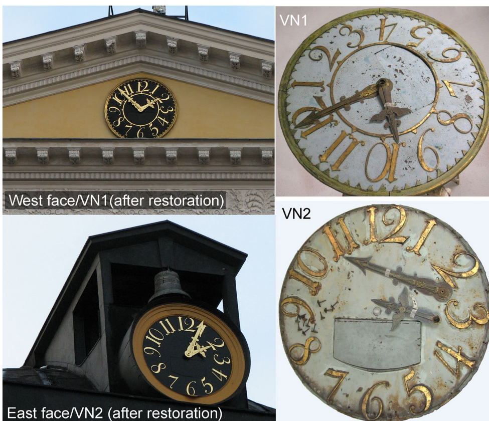
Fig. 1 Tower clock faces from the Government Palace in Helsinki before and after restoration works, west face/VN1 on the top and east face/VN2 on the bottom. Both clock faces were restored to have their original black colour
