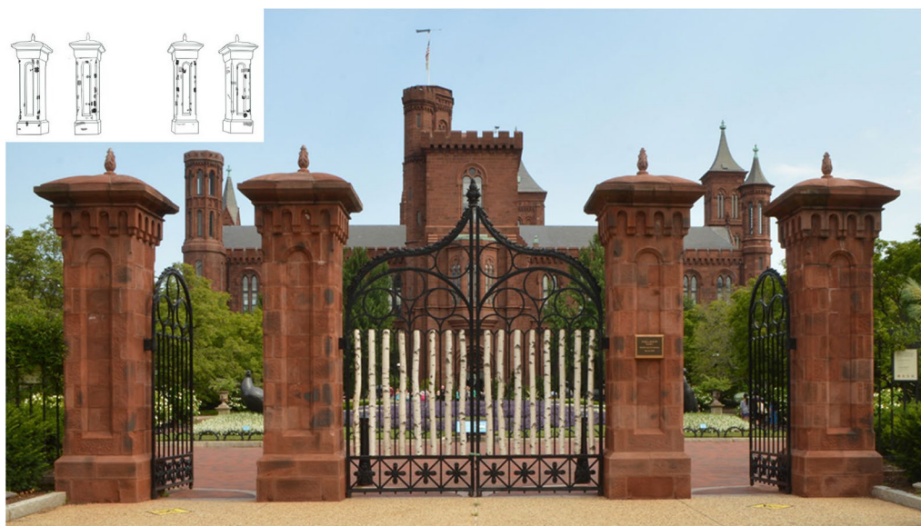
Fig. 2 Enid A. Haupt Garden gateposts with the Castle in the background. Inset: drawing depicts locations of rock varnish on the gateposts
