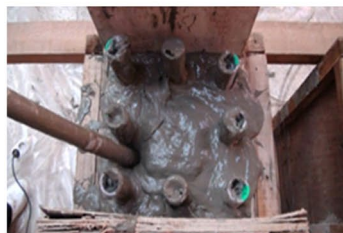
e Placing of HDFC
