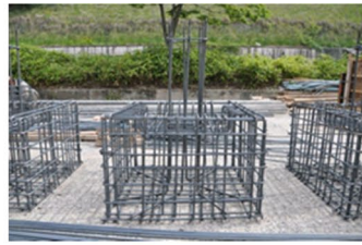
a Reinforced footing
