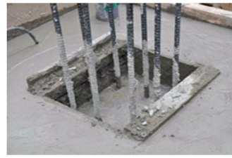
b Footing with precast box seat
