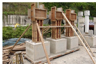
i Formwork of column
