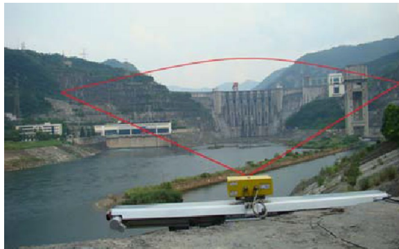
Fig. 6 IBIS-L equipment and the scenario from the radar point of view
