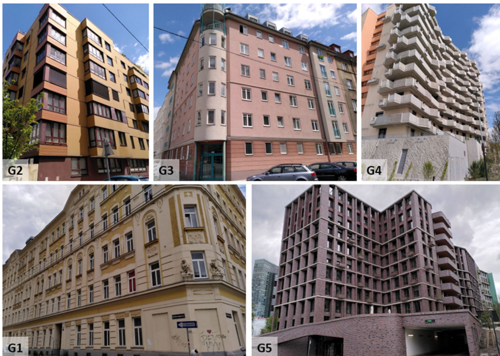
Fig. 2 Typical Viennese building types for the implementation in uhiSolver: G1 = Gründerzeit building, G2 = reinforced concrete building of the 1970s, G3 = hollow brick building of the 1970s, G4 = new reinforced concrete building, G5 = new high-rise brick building
